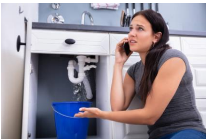
leaking of utilities & drainage
