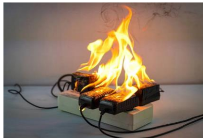
Overloading of electrical circuits
